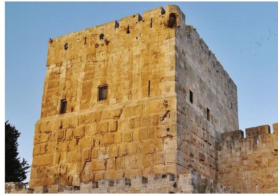
House at the side of a wall
